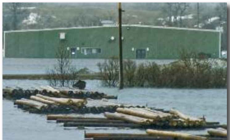
While flood waters reached KEM Electric Cooperative's pole yard, the poles were salvaged.
