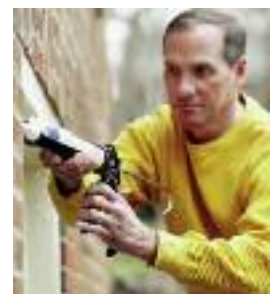
Simple weatherization steps, like caulking windows, will save money.
