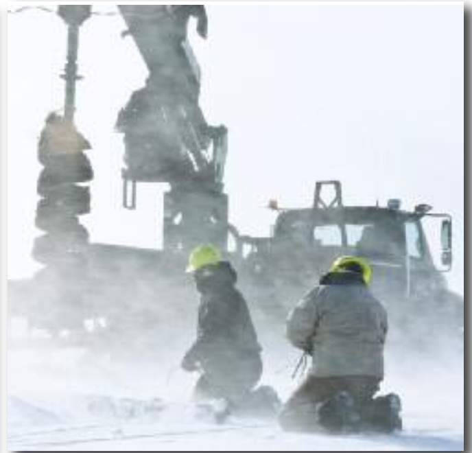
KEM Electric Cooperative replaced 988 poles during the restoration.
