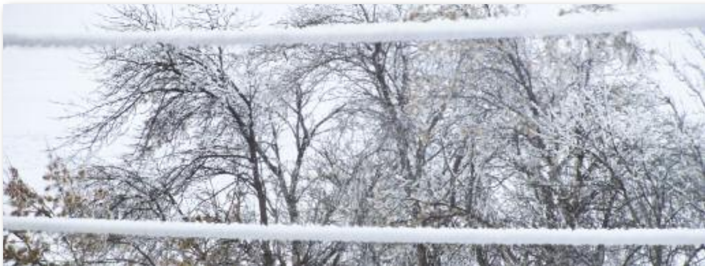
The frost and ice gripping the line accumulated over several days.
