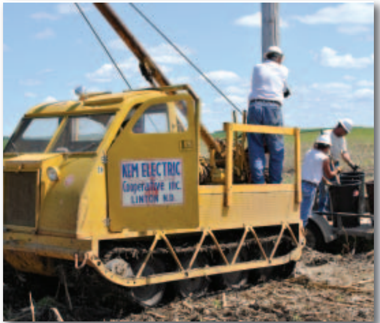
Lineworkers Dave Twardoski, on the ground by trailer, Tim Dockter, on the trailer, Jake Zink, driving the tracked vehicle, and Paul Hewitt, on the tracked vehicle, prepare to straighten out one of six transmission poles that were pushed because of the high winds.
